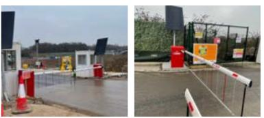
The SOSEC, INSTABOOM and Wireless GS6 barriers are all fully mobile and can be moved easily when the site requires, meaning no wires or cables. They were delivered ready to work and are up and running in minutes.
