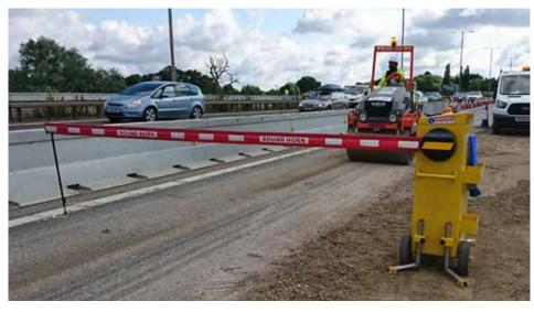
the monotonous and dangerous job of manning a barrier-guard to be done automatically. Reducing the number of operatives having to stand in the line of moving traffic to protect work crews further down the lane by providing a physical remote barrier, stopping unauthorised vehicles entering an active construction area. INSTABOOM® has dramatically reduced the sites' PVM budget and redeploying staff to more productive work.
