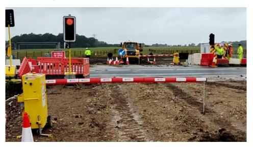
Always ready to solve a one-off problem, the Solar Gates UK technical team integrated the Highways England award winning, solar hybrid, INSTABOOM® barriers to a standard traffic signal crossing system. The resulting combination ensured the INSTABOOM® barriers held haul route traffic until the traffic signals had closed the live lanes and the haul route signals were green.
