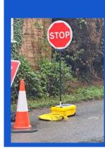
Deploy Traffic Management set up, according to required standards. Set Stop/Go poles in place and sandbag handle if conditions require.
